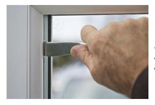
To ensure that your window is suitable, slide a butter knife into your rubber gasket and push it as far as it will go. To help the knife ease in, you can use washing up liquid or furniture polish.
