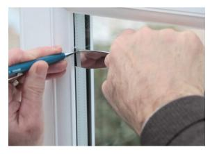
Mark the distance the blade travels under the gasket.
