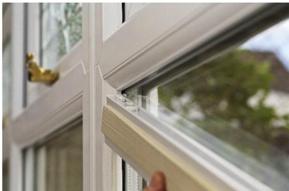
To fit the blind, slip the tab on the top rail of the blind in between the glass and the rubber gasket. Again, you can use washing up liquid or furniture polish to make the procedure easier and to avoid damaging your window.
