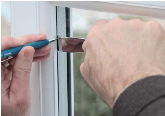
Mark the distance the blade travels under the gasket.
